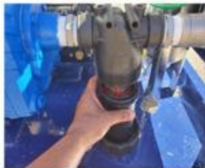
Pull down case with Strainer
