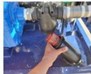
Remove all components for Inspection
