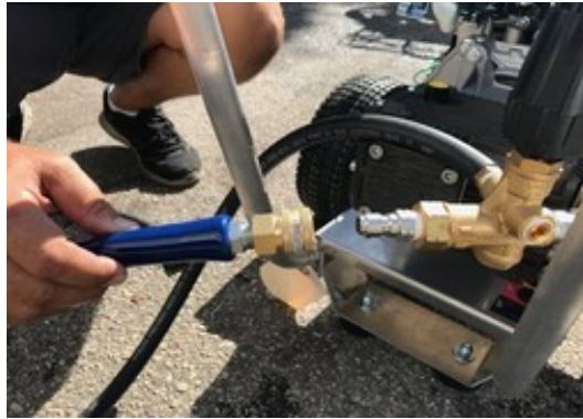
Figure #6 - Connect HP Hose to the quick connect under pressure regulator
